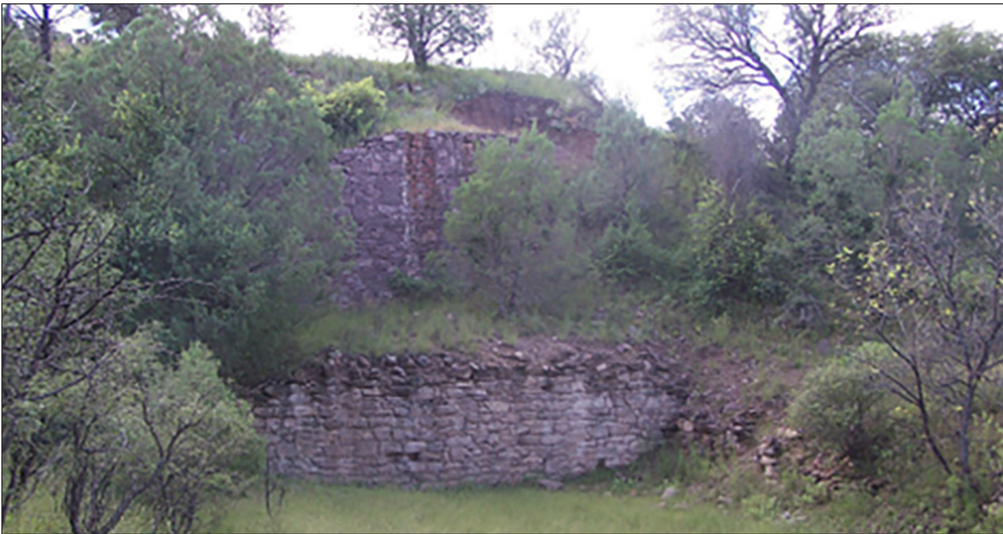
Terraced retaining walls
