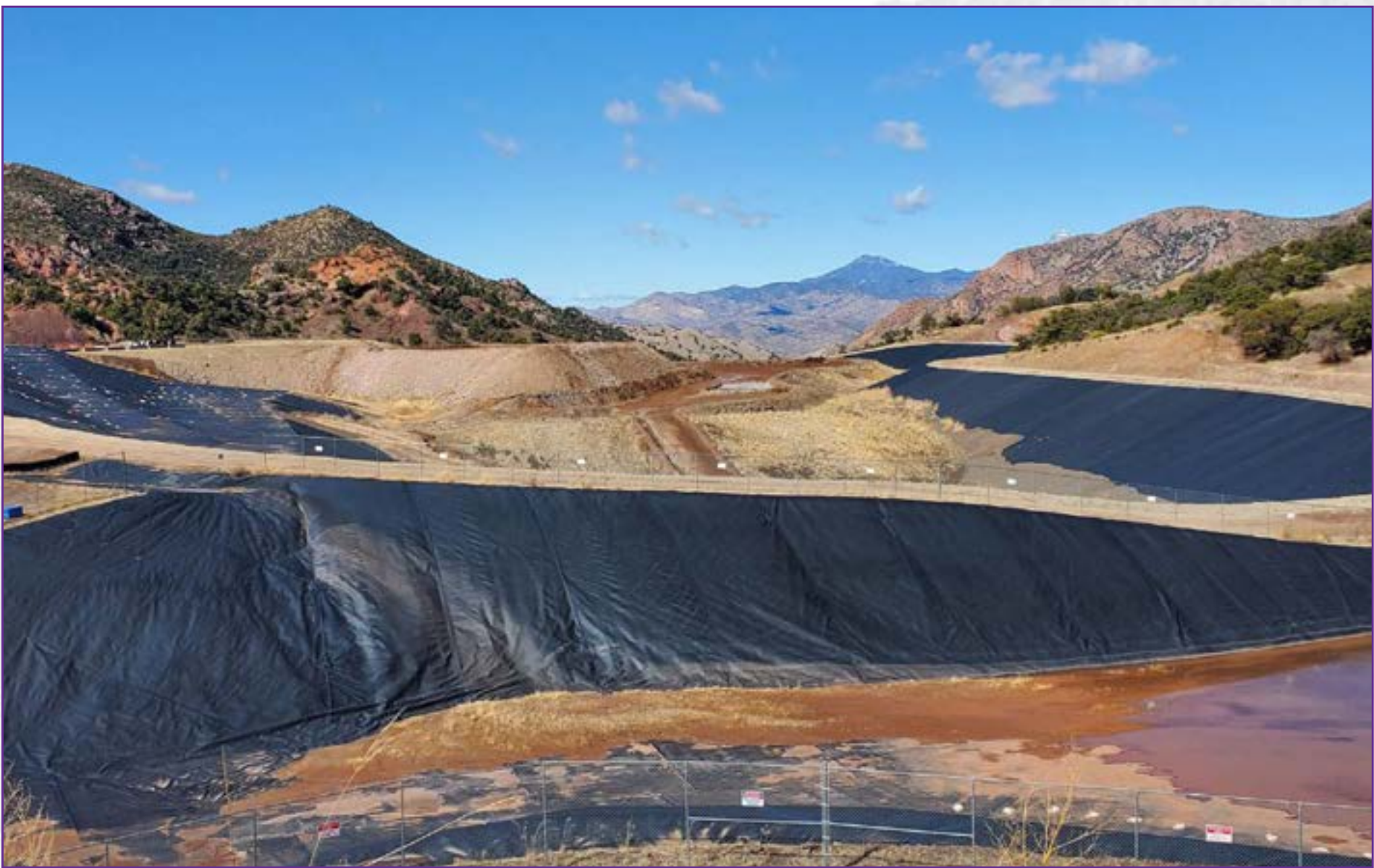
Dry Stack Tailings Facility (TSF1) on South32 Hermosa private land.
